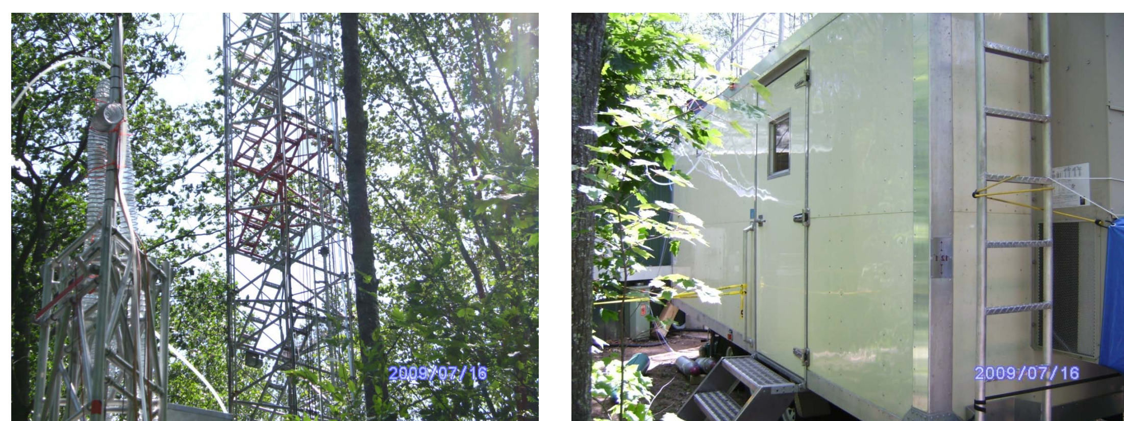
CABINEX Tower and trailer inlet. MACL
